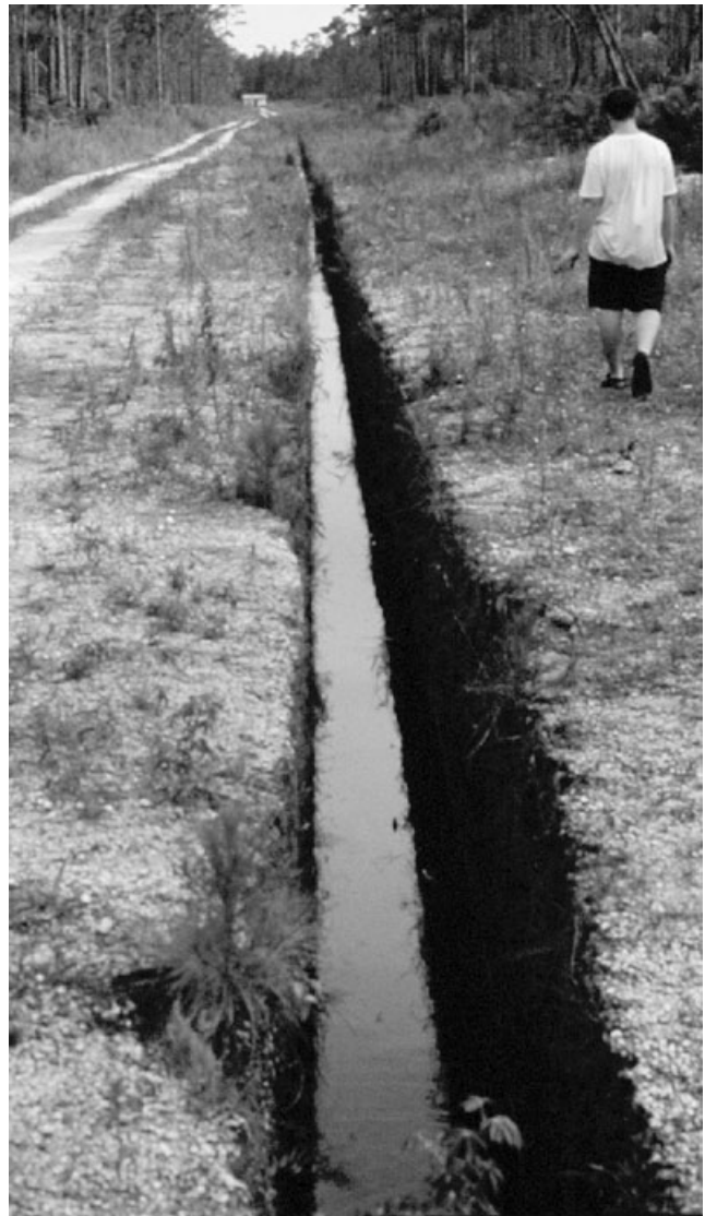
Figure 1. One of four trenches radiating from a central pump (in building in the distance) that makes up a typical freshwater well on North Andros. Note the narrowness of the trench and the vertical walls that exclude terrestrial predators. Each trench is ~2 m deep.
